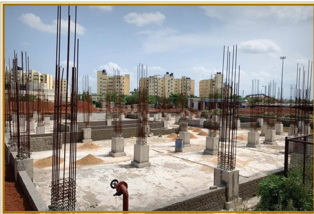
Ongoing Construction of Trauma Building
