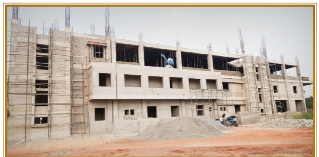
Ongoing Burn unit Construction funded by NTPC.
